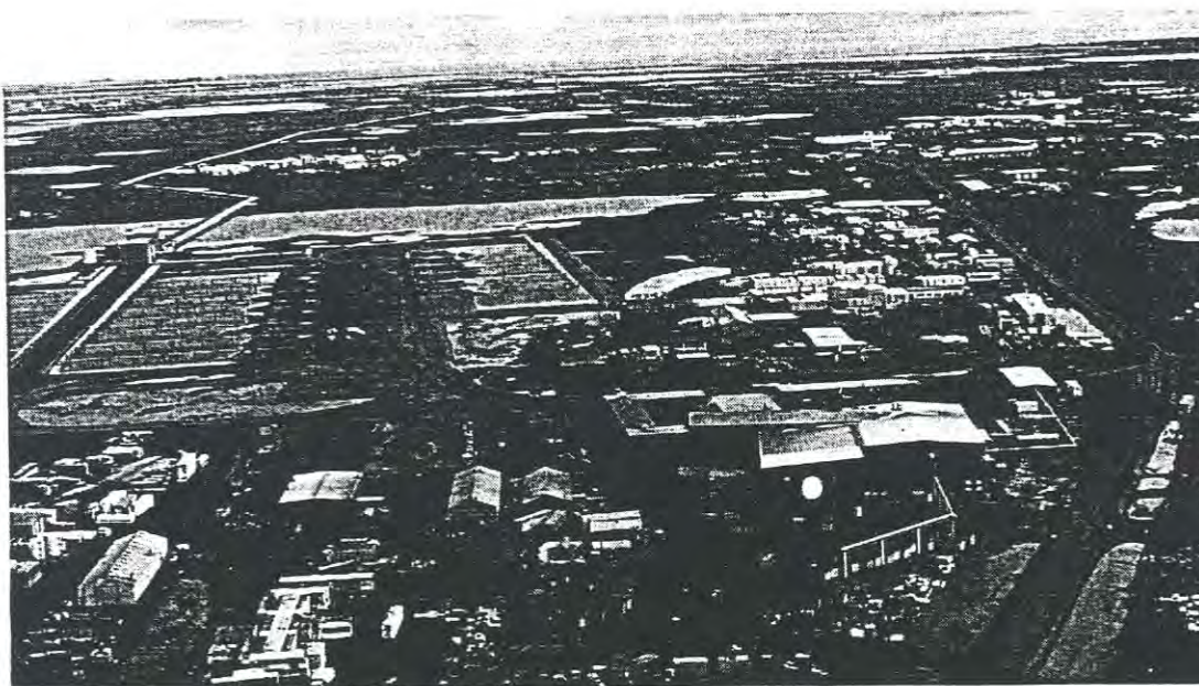
Figure 3. A portion of the Prudhoe Bay Oil Field including networks of pipelines, roads, and gravel pads. The large rectangular gravel pad on the left side is a drill site with 14 well heads and two reserve pits. Complex cumulative impacts are associated with such large developments.
