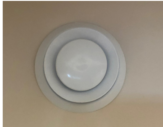
Figure 15. Example of a Fresh 80 System Installed on a Wall. (NREL, 2022)
