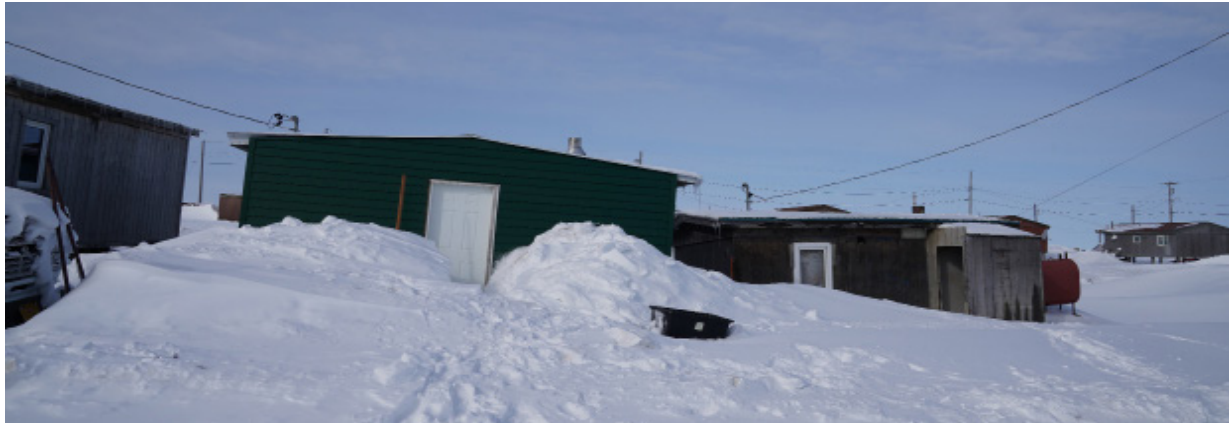
Figure 3. Point Lay Home Tilting. (NREL, 2022)
