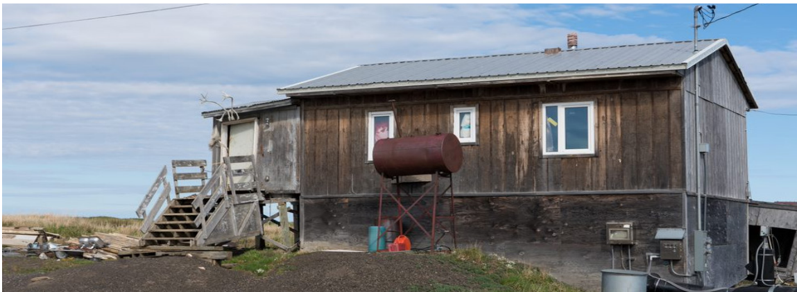
Figure 24. Example of Porch Conditions. (Point Lay Resident Bill Tracey, 2022)
