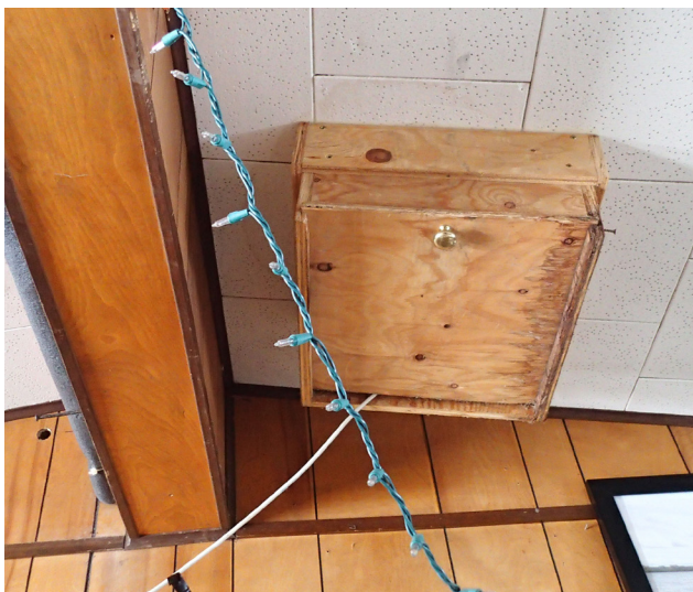
Figure 16. Example of a Kingaq Installed on a Ceiling. (NREL, 2022)
