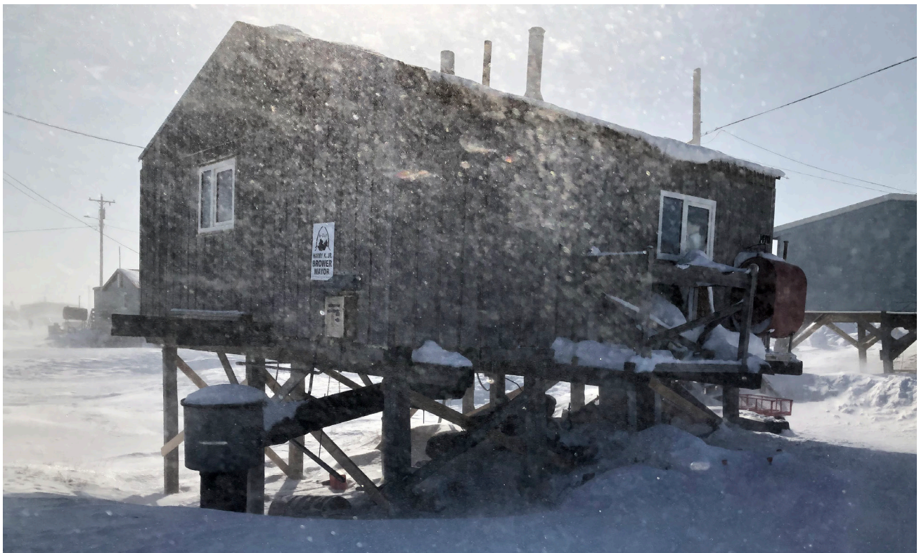
Figure 5. Point Lay Home Atop Pile Foundation. (NREL, 2022)
