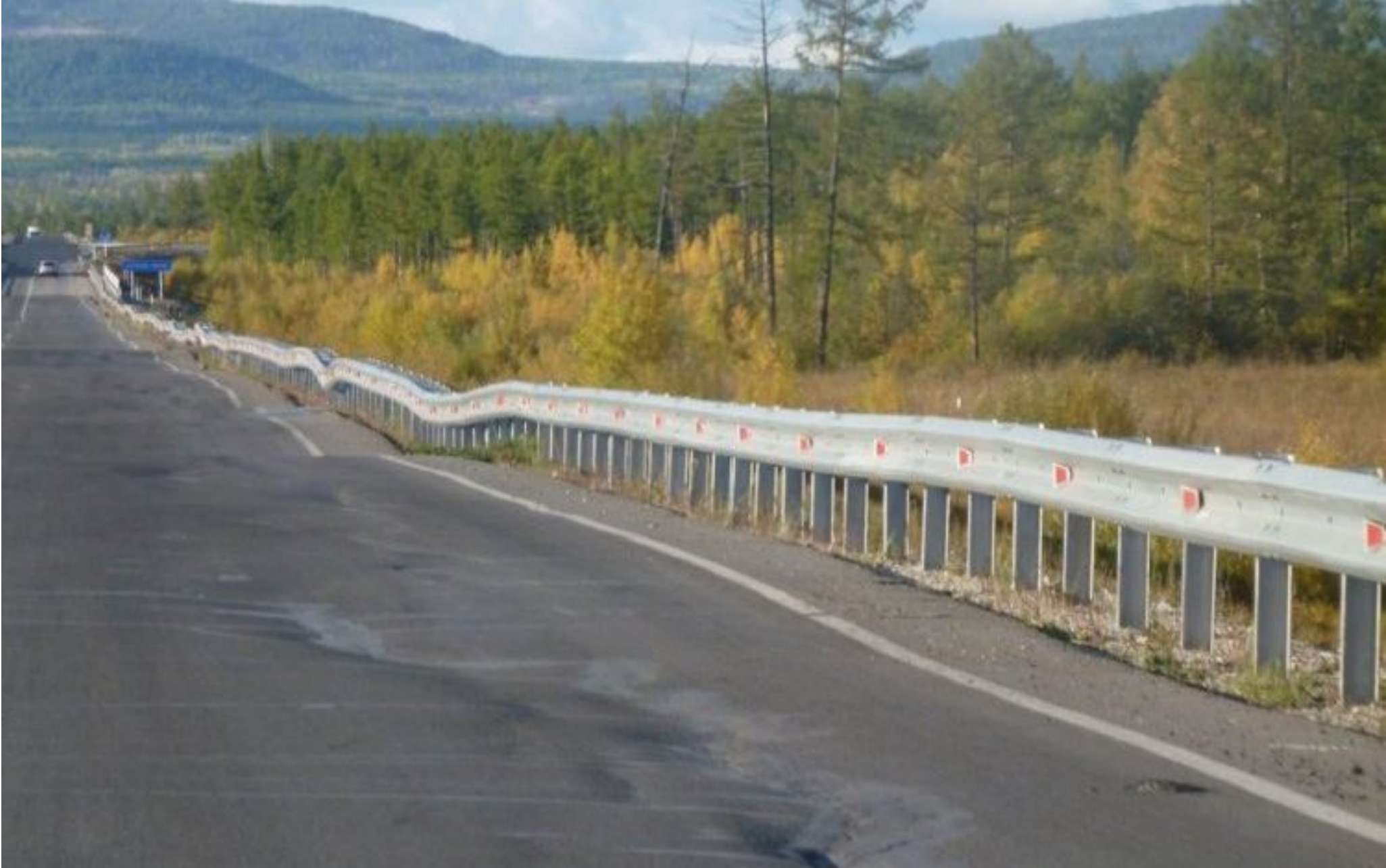
Amur Highway after reconstruction in 2010
